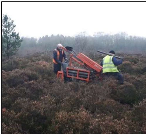
Photos 5.2-1a and 5.2-1b. Mobilisation and set-up of rig across concealed drains and woodland made piezometer installation a challenge.
