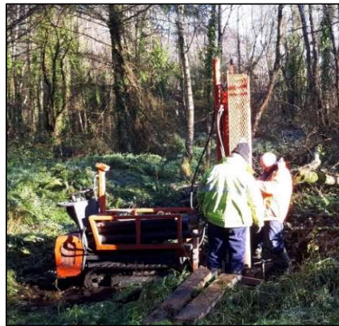
Photos 5.2-1a and 5.2-1b. Mobilisation and set-up of rig across concealed drains and woodland made piezometer installation a challenge.
