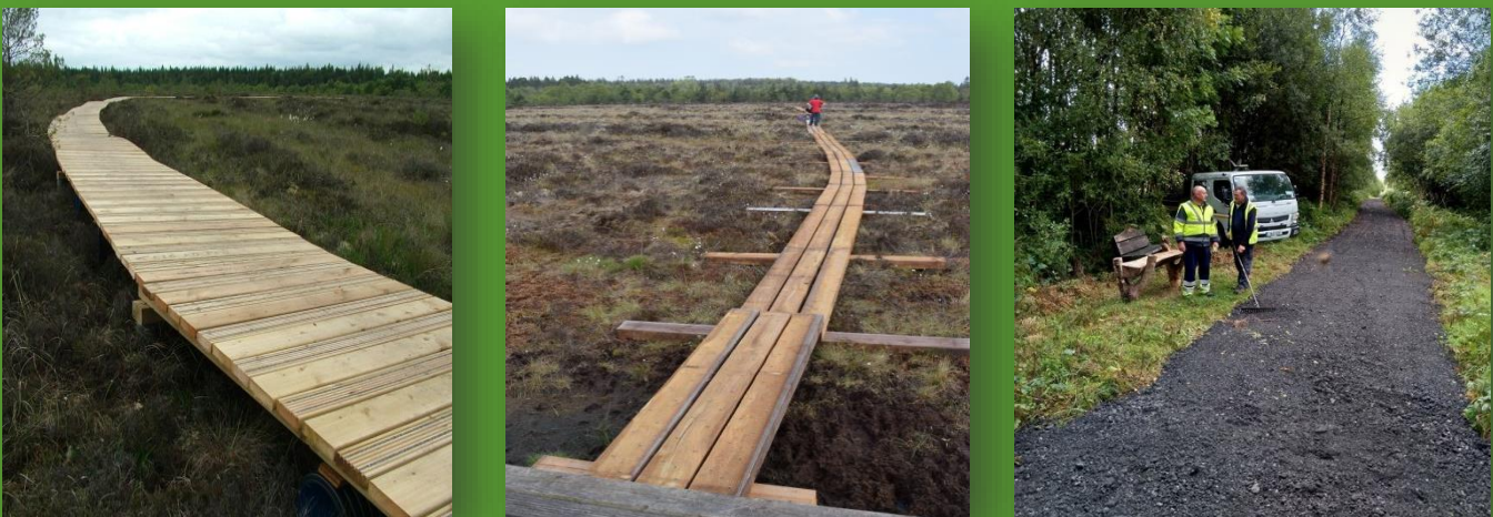
Figure2: Boardwalk (left), Bog-bridge (middle), Path with planings (right). Source: Abbeyleix Bog Project
